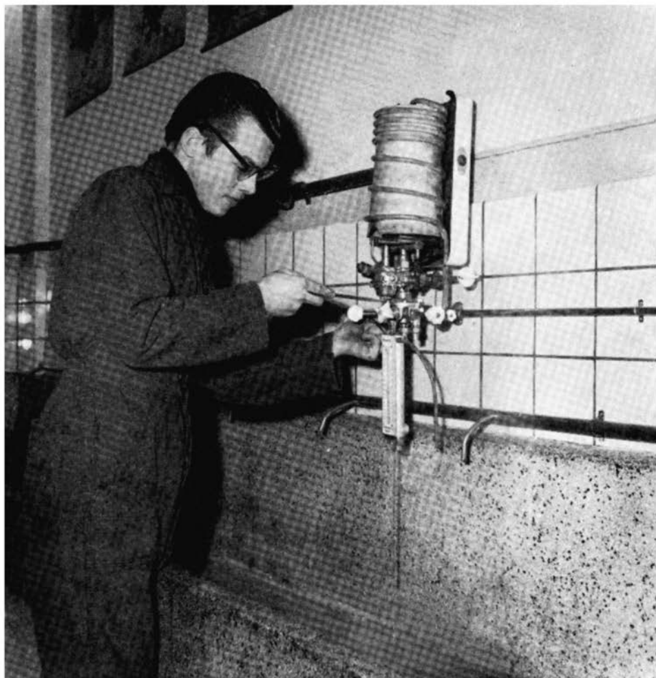
Afd. Fitten: geysir controle
